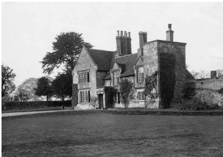
Temple House on the Arbury Estate earlier inhabited by the Knights Templar
